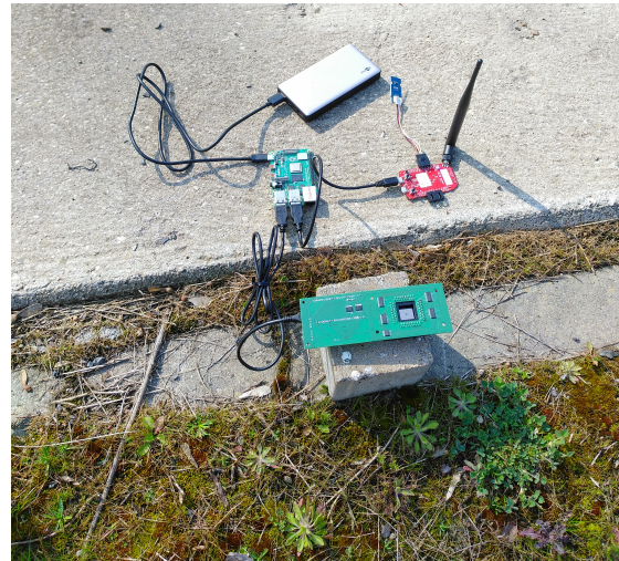
Fig. 2: A wireless sensor node integrating an array of nanosensors for toxic gas detection and a Raspberry Pi and the Zolertia platform for network management.
